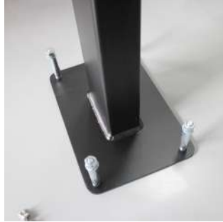
2. Drive in the expansion screws
